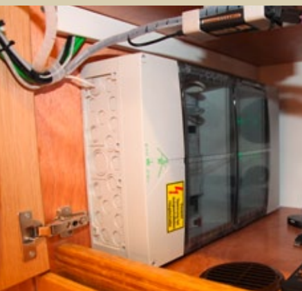
Ventilated, rubberized KNX® interface and line sub-distribution
