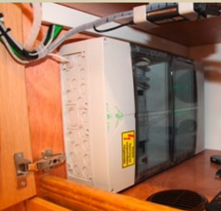
Ventilated, rubberized KNX® interface and line sub-distribution
